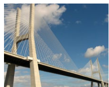
Vasco da Gama Bridge (PT)
