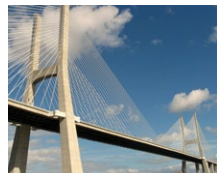
Vasco da Gama Bridge (PT)
