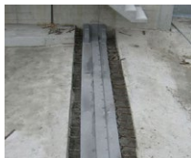
Joint prior to concreting
