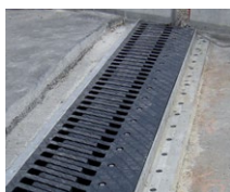
Sliding finger joints
