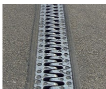
Cantilever finger joint
