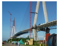
Can Tho Bridge (VN)
