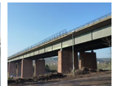
Lautertal Bridge (DE)
