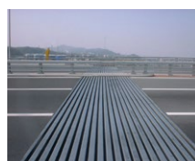
Modular expansion joints
