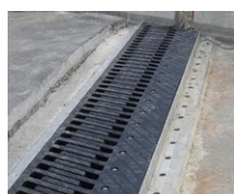
Sliding finger joints
