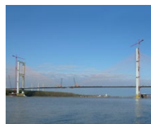
Audubon Bridge (USA)
