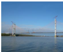
Audubon Bridge (USA)
