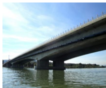
Traismauer Bridge (AT)
