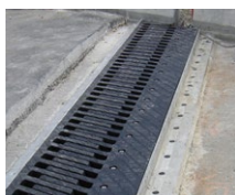
Sliding finger joints
