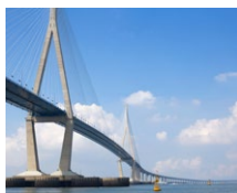
Incheon Bridge (KR)
