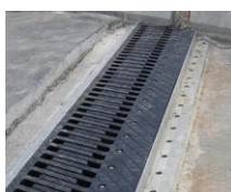
Sliding finger joints
