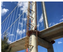
Longjiang Bridge (CN)
