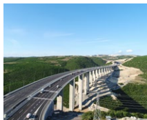
Liman Viaduct (TR)
