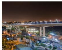
Chilina Bridge (PE)
