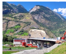
A9 motorway – Raron (CH)
