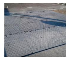
Mini-Flyover Type A can be used to cover the entire road or just individual lanes, e.g. in a 3+1 traffic routing.
