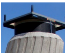
Elastomeric bearings
