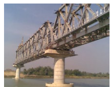
Bhagirathi Rail Bridge (IN)
