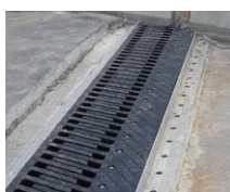
Sliding finger joints
