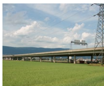
Viaduct Yverdon (CH)
